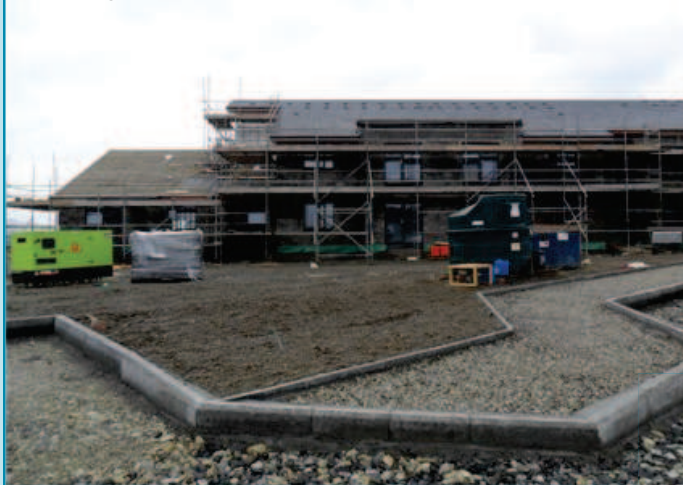
Mull Progressive Care Centre under construction
